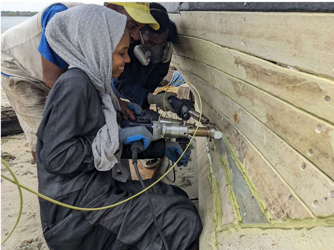
Boatbuilder Nuru, welding and sealing planks on the Flipflop taxi dhow
